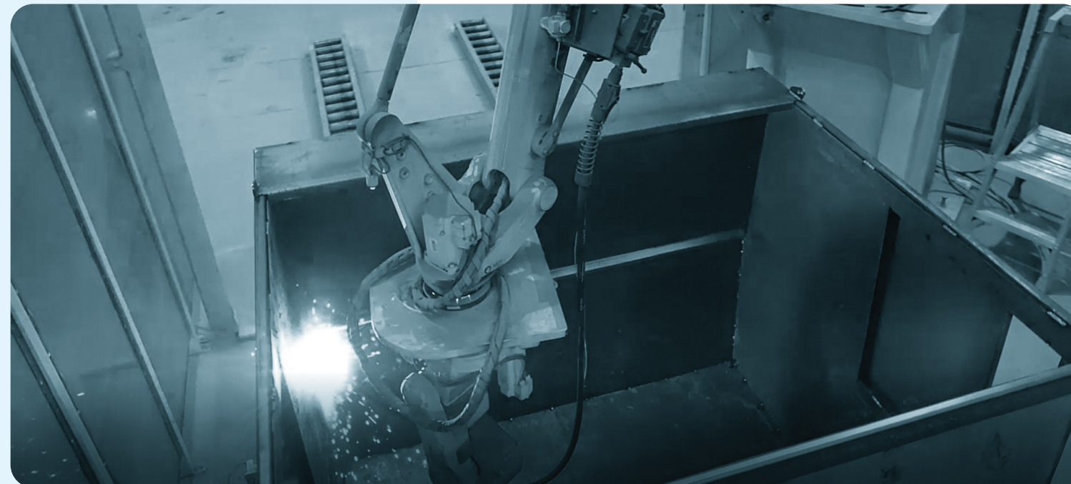
Automation of FEL line in Eagleville, TN facility.
